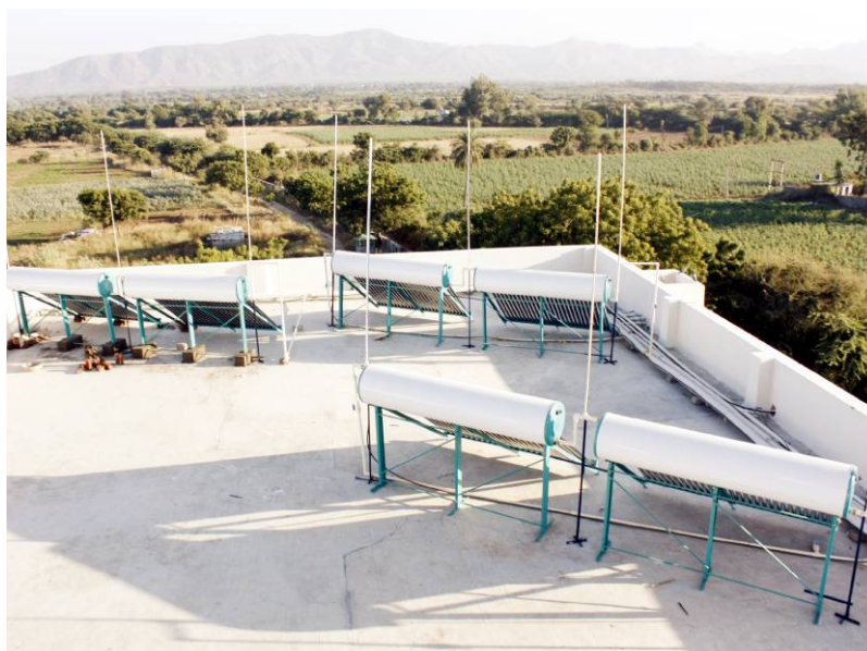
Solar panel installation on the roof of the nursing students hostel
